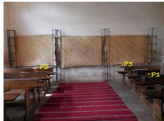
**Fig 5:** Classroom with panels mounted on the rear wall and coir mat laid on the floor
